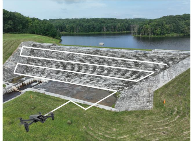
Fig. 1. Downstream slope of the Upper Deckers Creek dam (WV, U.S.A.), the Parrot Anafi USA Gov drone used in the experiments of this paper, and an example of a dam inspection trajectory specified using the requirements of the mission.
